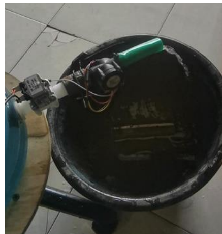
Figure 6. Flow Meter Measurement on Water Pipes
